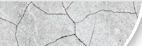
CPMF4149 - Cracked Concrete
