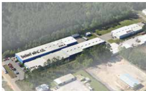
Aerial shot of Denny Manufacturing Co., Inc.
